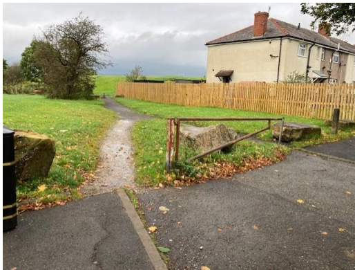
Photo 2: Public Right of Way No 82
